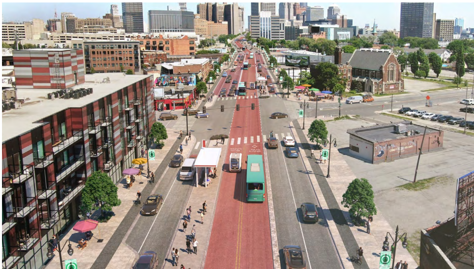
Figure 44. The preliminary design of the Detroit Mobility and Innovation Corridor, which was awarded $25 million by USDOT in 2022. Image Credit: City of Detroit
