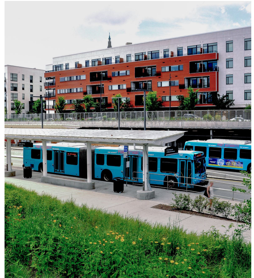
Figure 12: The East Liberty TOD along the Martin Luther King Jr. East Busway in Pittsburgh, a bus-only highway that operates BRT service. The TOD project improved bus stops, created 360 housing units and 361 jobs, and increased ridership at the bus station by six percent. 18 Image Credit: Pittsburgh Regional Transit.
