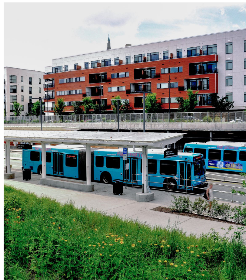
Figure 11: The East Liberty TOD along the Martin Luther King Jr. East Busway in Pittsburgh, a bus-only highway that operates BRT service. The TOD project improved bus stops, created 360 housing units and 361 jobs, and increased ridership at bus station by six percent. 2 Image Credit: Pittsburgh Regional Transit.
