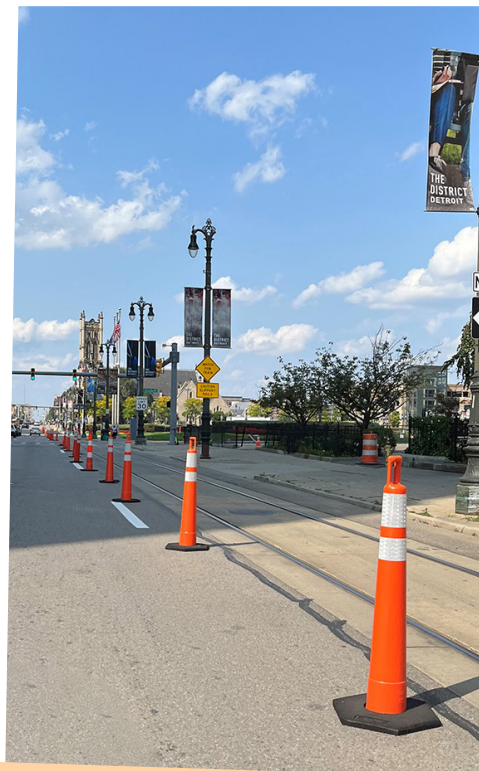
Figure 6: QLINE's tactical transit lane pilot on Woodward Avenue.
